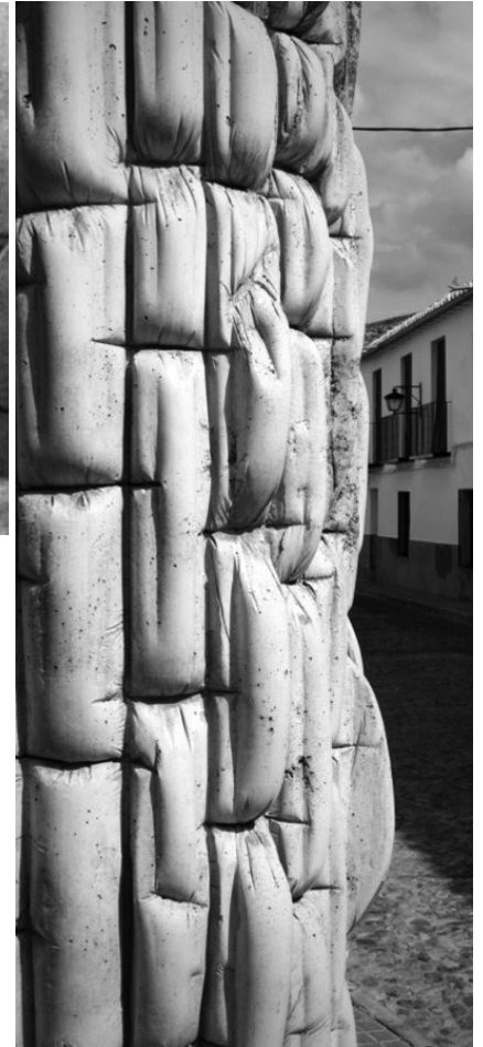
Frei Otto soap bubble model (top left), Antonio Gaudi gravity model (bottom left), Miguel Fisac fabric form concrete wall (right)
