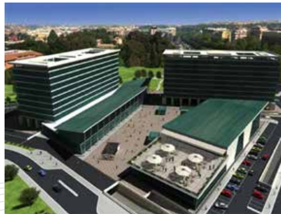
Image 2.9: This is the rendered version of Centro Navigatori. This is what it could have looked like. Notice the green space behind the buildings (Image from Catarci, 2013).
