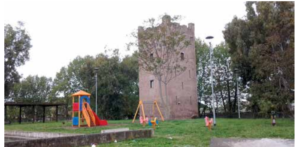
Image 2.1: Image of Tor Marancia Tower (Image courtesy of Roya Sabri).
