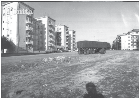
Image 2.5: Construction in Tor Marancia (Image from l'Unità).
