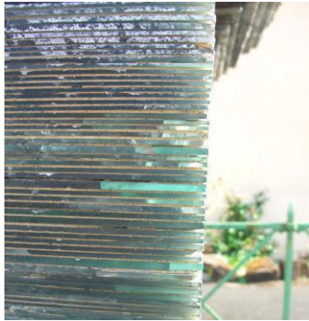
Left: detail of the pedestal of La Croix des Verriers (the glassmakers' cross) in Boisses-Penchot, Aveyron, France, 1861, showing the stacked sheets of glass construction. Middle: Detail of connection between the steel glass-holding frame and the exoskeletal primary steel column in Mies van der Rohe's Farnsworth House, 1951. Right: Detail of the clamp fitting securing 4 sheets of glass in the Juilliard Alice Tully Hall, NYC, 2008, Diller Scofidio +Renfro Architects.
