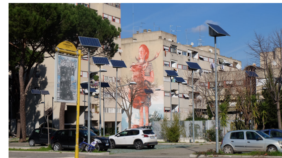
Figure 5.31: Public housing complex forms a district
