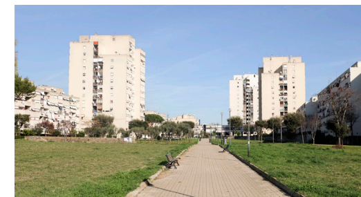
Figure 5.6-8. Public housing complex in Torreviecchia
