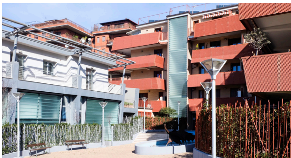
Figure 5.20. Palazzine in excellent condition scored 3
