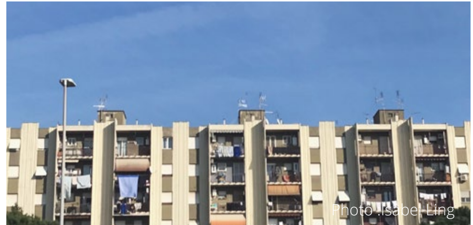
Fig 18: Public Housing in Torre Maura
