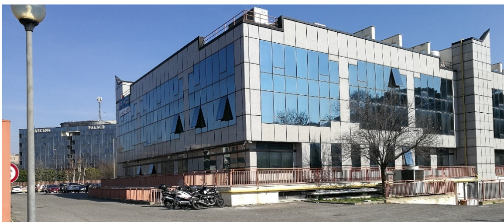
Figure 10: Low Rise Office building on Via Attilio Benigni.
