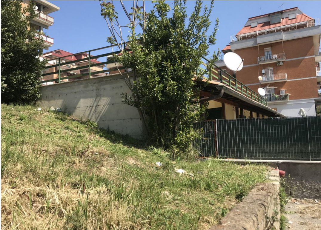
Figure 9: Building northwest of gate, negotiate with owner
