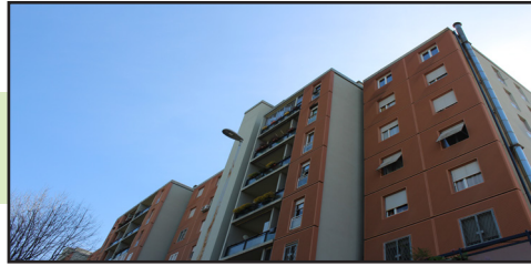
First building of Colli Aniene completed, established as a construction cooperative legalized by Law 167
