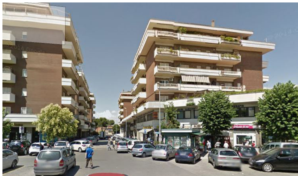
Figure 49. Current parking area in front and between Blocco Stecca
