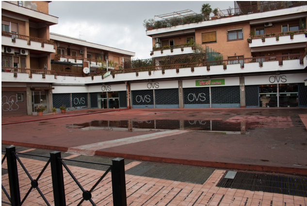
Figure 11.4.1 Existing OVS Complex conditions
