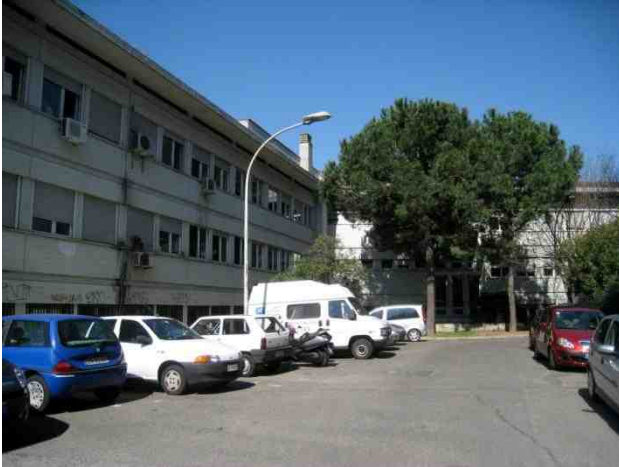
Figure 30. Clinic – “Sanitaria Locale”, Entrance on Via Cartagine. Photo by Dennis Tejada.
