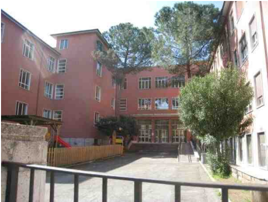
26. Primary School Salvo D'Acquisto, Via Selinunte Figure 23-27 Photographed by Dennis Tejada.
