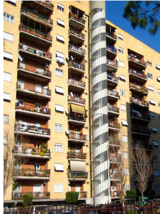
Building in the Northwest District. Photo credit: Cassandra Gallagher
