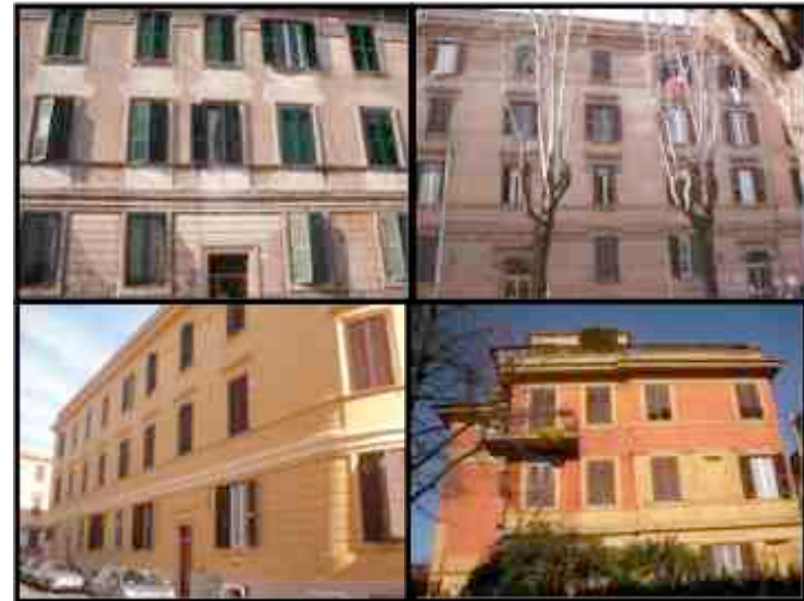
Type 2: Three-story Apartment Buildings Covered with Stucco
