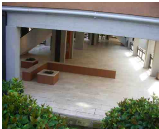
Figure 2: 13: Residential structure (Ni, 2009)
