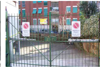
Figure 2:62: Fenced in area (Osho, 2009)
