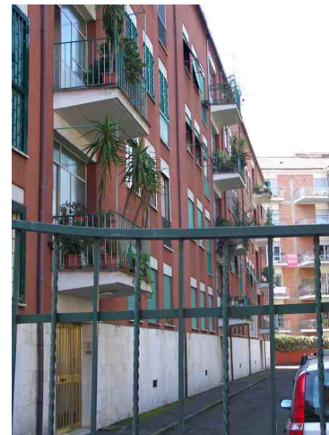
Figure 2:63: Fenced in area (Osho, 2009)
