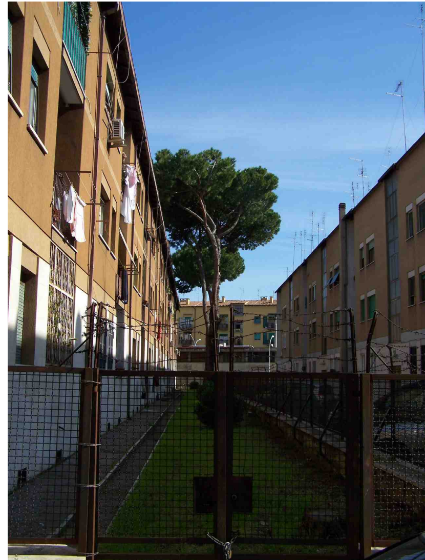
Figure 2:58: A typical private street, fenced off from the main public street, with street trees, parking spaces, sidewalks and overlook from adjacent blocks. (Osho, 2009)
