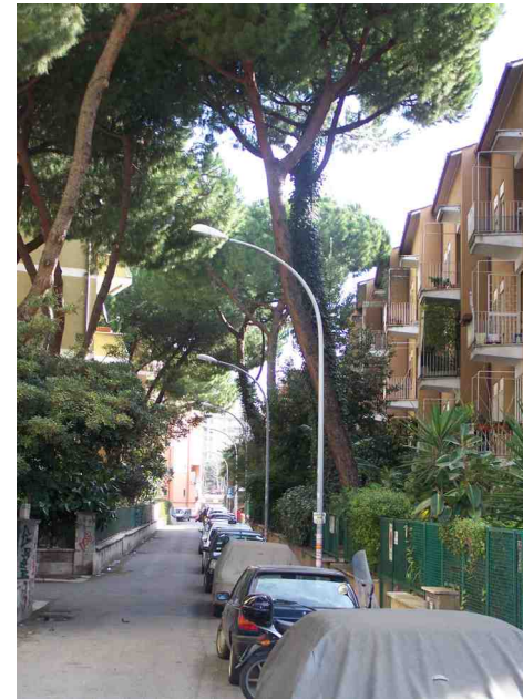
Figure 2: 47: Via Jerapoli's beautifully green mid-rise buildings, dotted with ample private balconies (Osho, 2009)
