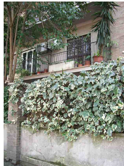
Figure 2:11: Residential structure (Ni, 2009)
