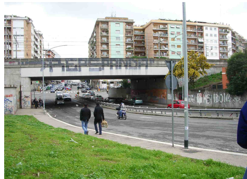
Figure 2:17: Looking East on Via di San Paolo (Ni, 2009)
